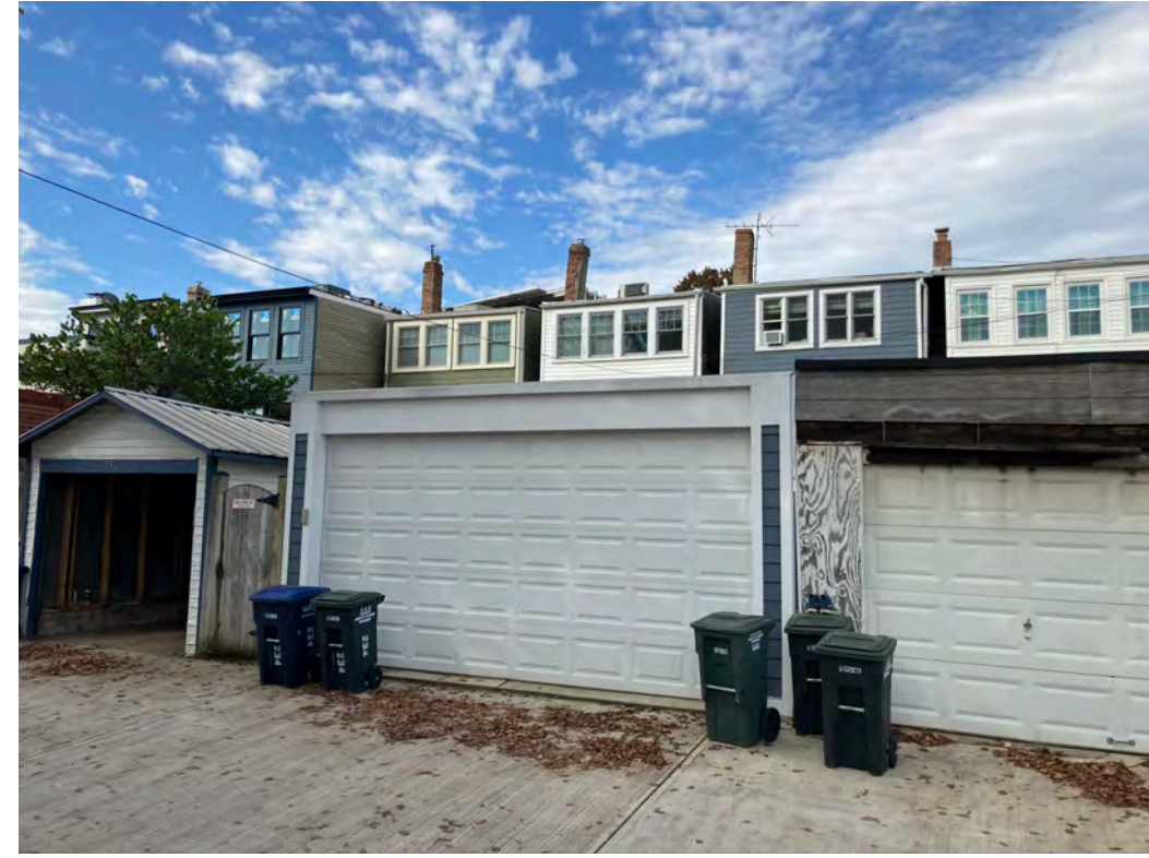
ALLEY NORTH VIEW
