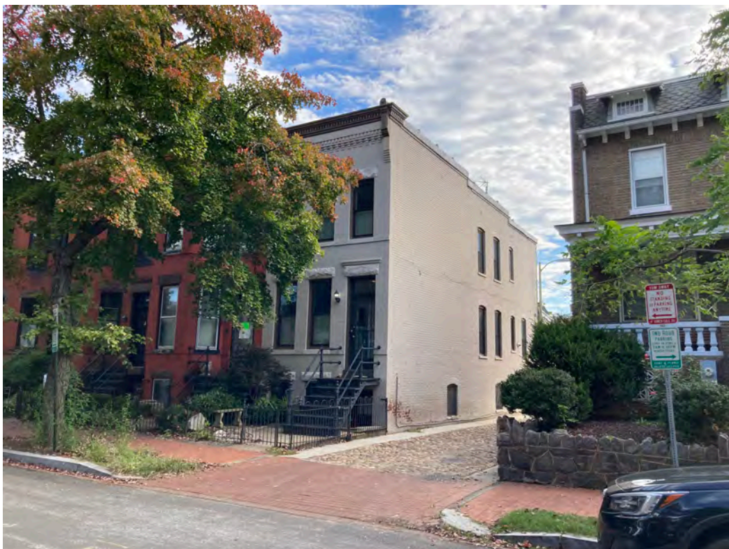
SOUTH VIEW, 10 TH STREET SE
