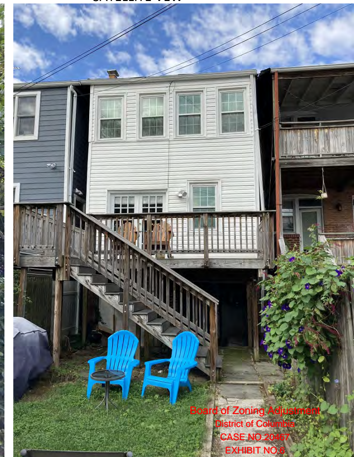
EXISTING REAR FACADE
